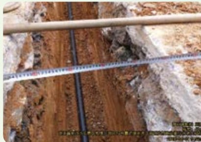
The pictures provided by visualisation system - construction site of gas pipeline
