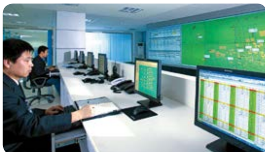
The dispatching and monitoring system can achieve real-time monitoring of the status of piped gas, customers facilities and heat distribution within the district.
